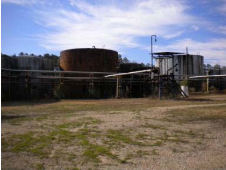
Figure 3. Large storage tanks
