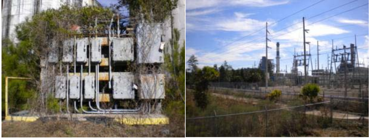
Figure 4. Potential electrical connection points
